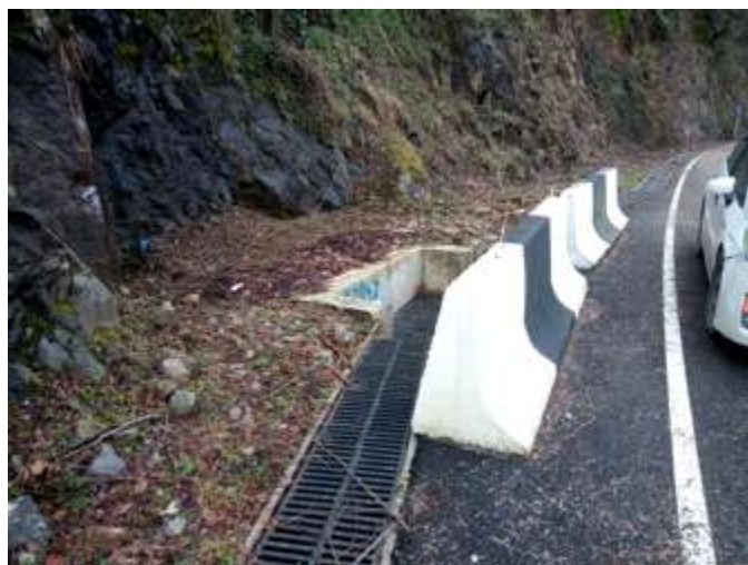
KM 0+409 Installation of Pipe
