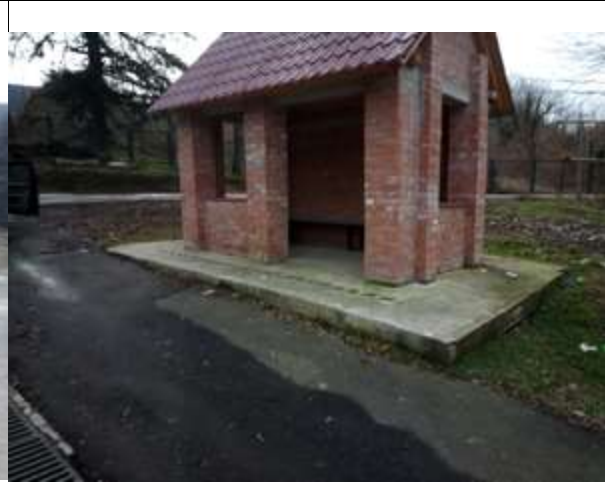
KM 14+822 Construction of Bus Stop
