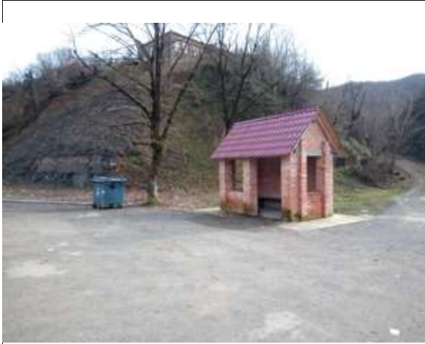
KM 2+467 Construction of Bus Stop
