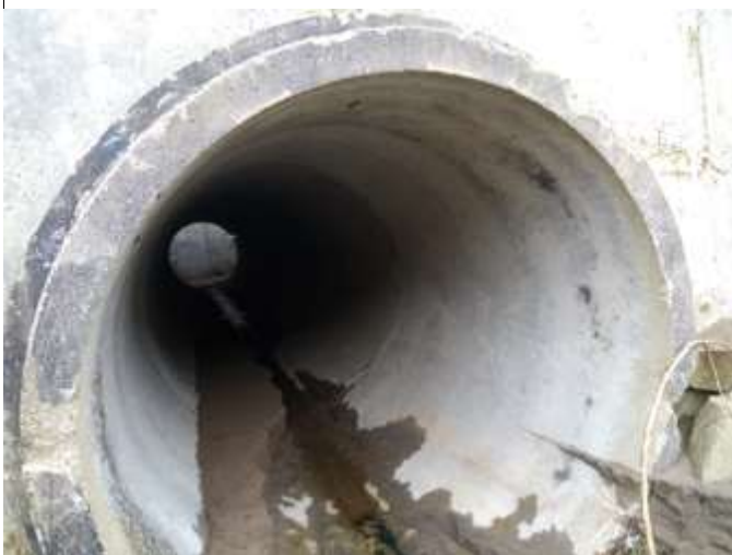
KM 6+428 Installation of Pipe.
